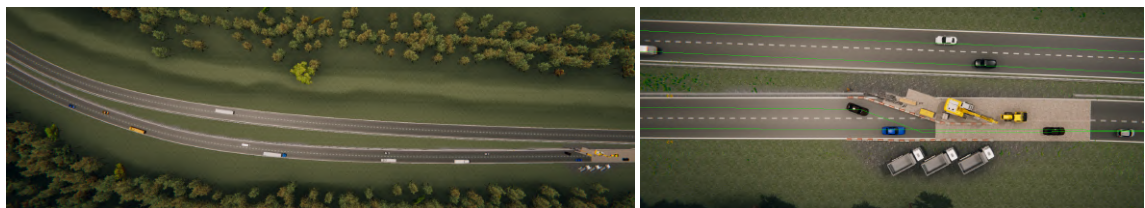
Fig. 2. Top down views on the construction site.
